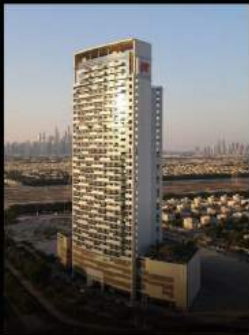
Al Jawahara Tower JVT, Dubai
