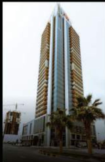
Al Manarah Tower JVT Dubai
